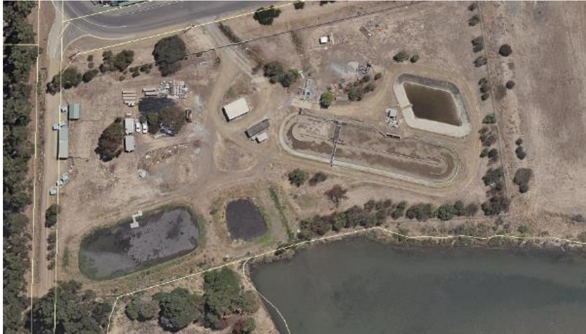
Figure 62-1: Sorell Sewage Treatment Plant
