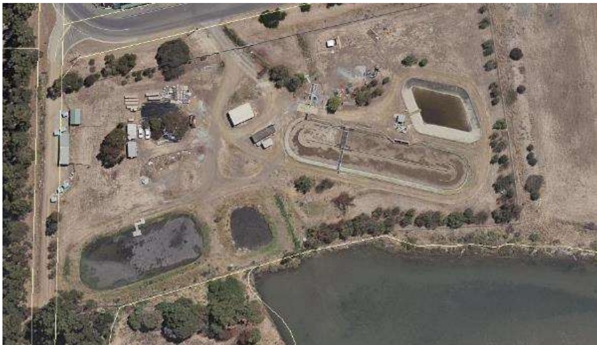
Figure 62-1: Sorell Sewage Treatment Plant
