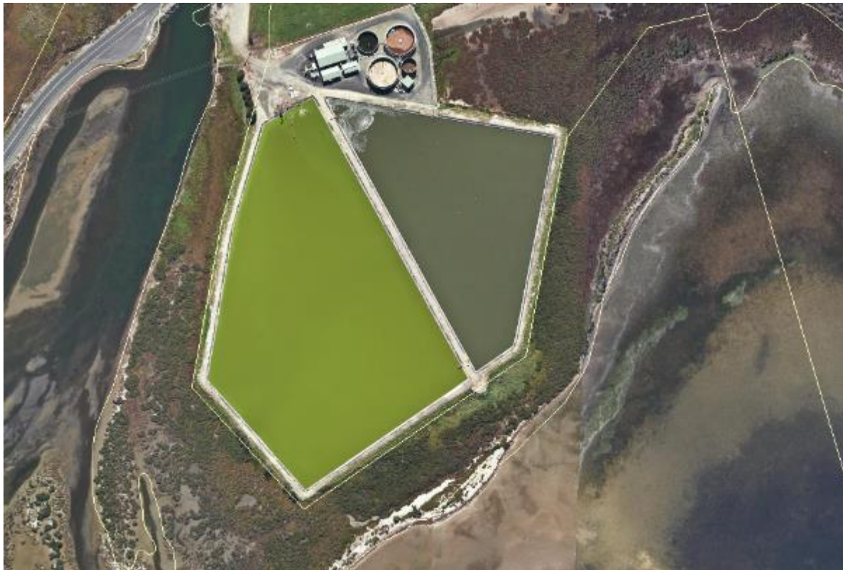
Figure 63-1: St Helens Sewage Treatment Plant
