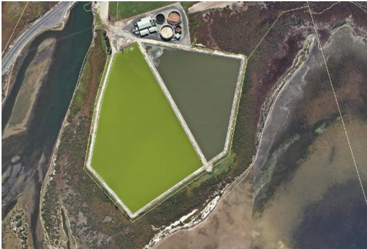
Figure 63-1: St Helens Sewage Treatment Plant
