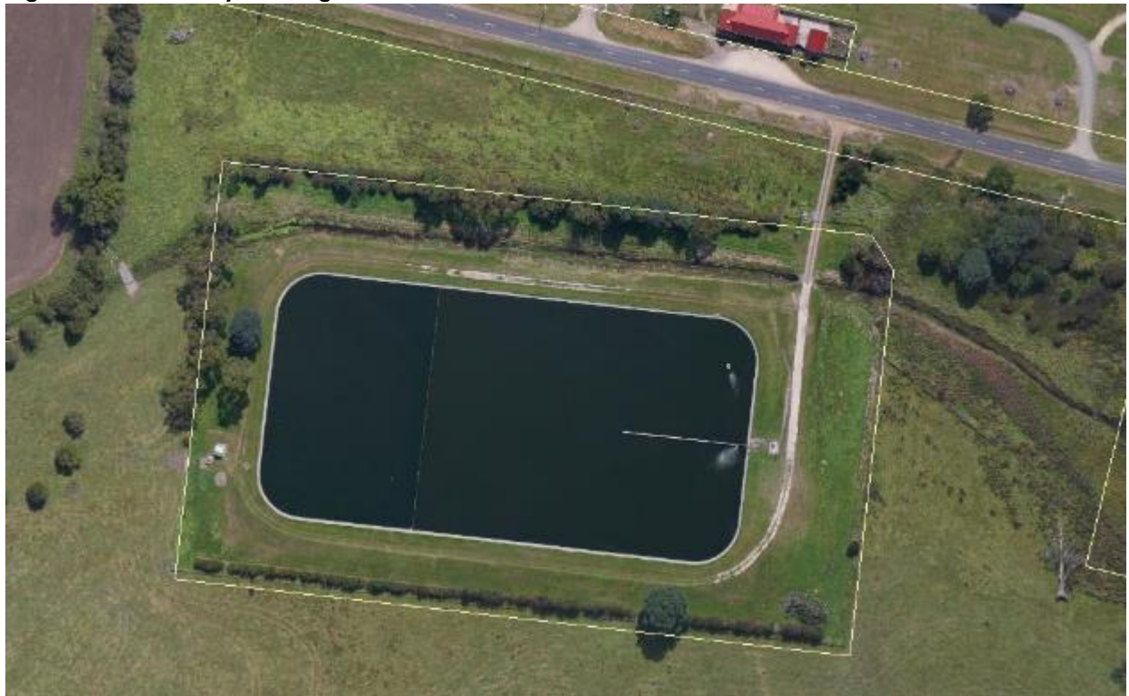
Figure 64-1: St Marys Sewage Treatment Plant
