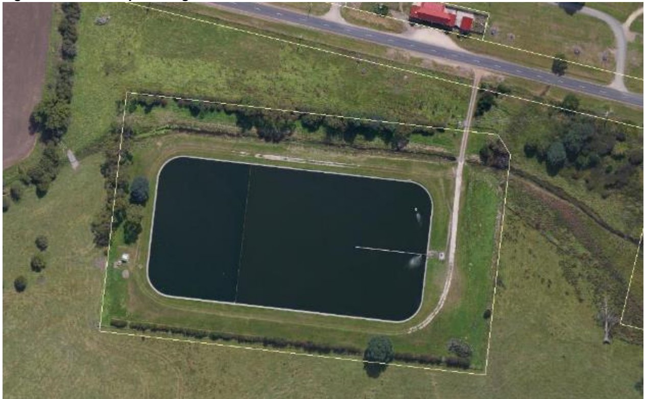
Figure 64-1: St Marys Sewage Treatment Plant
