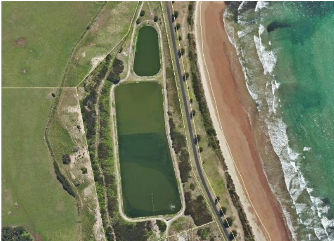
Figure 65-1: Stanley Sewage Treatment Plant
