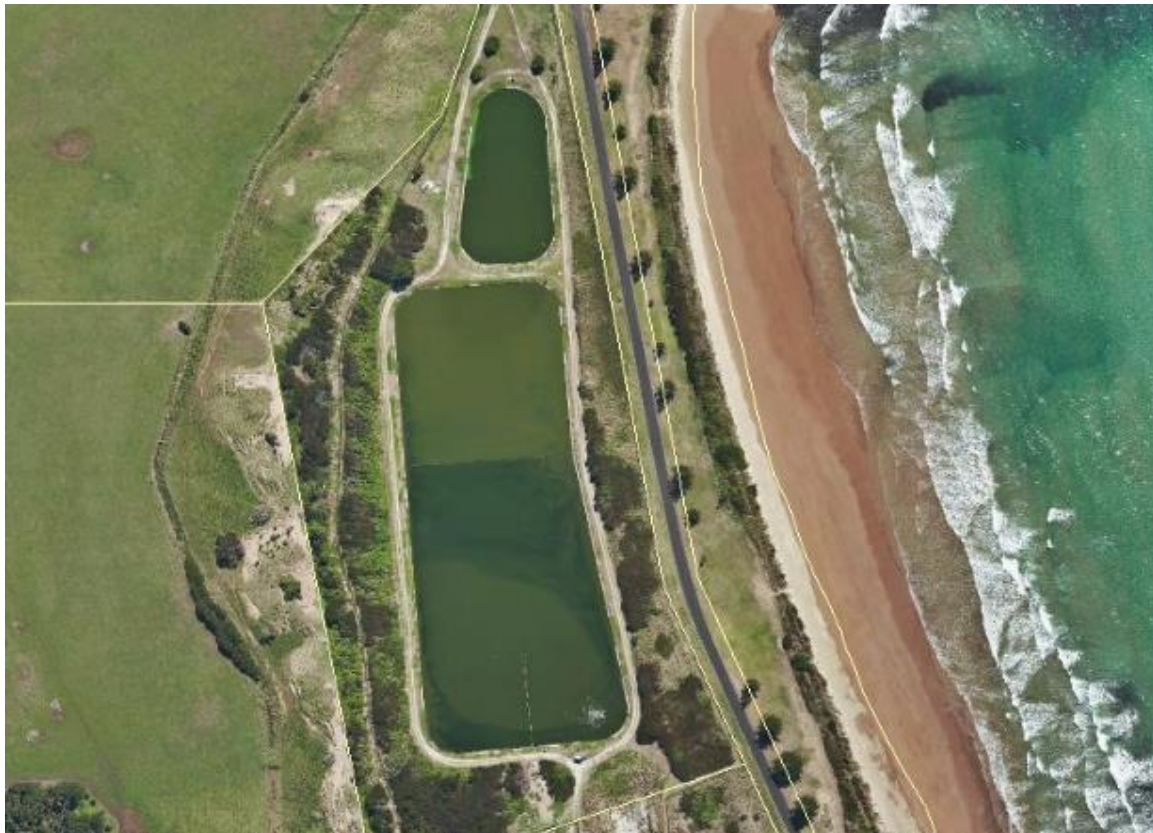
Figure 65-1: Stanley Sewage Treatment Plant
