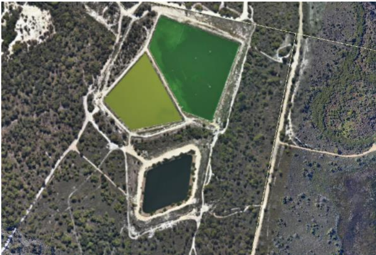
Figure 66-1: Steiglitz Sewage Treatment Plant
