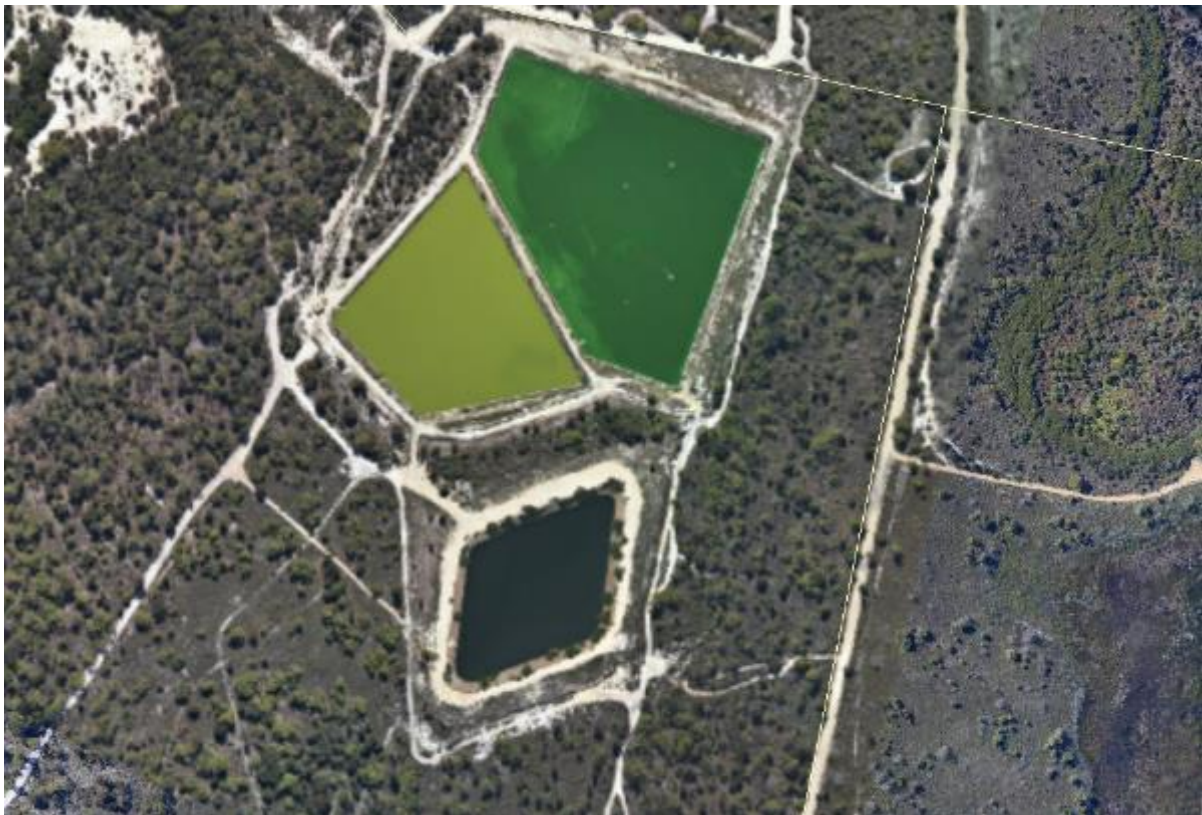
Figure 66-1: Steiglitz Sewage Treatment Plant
