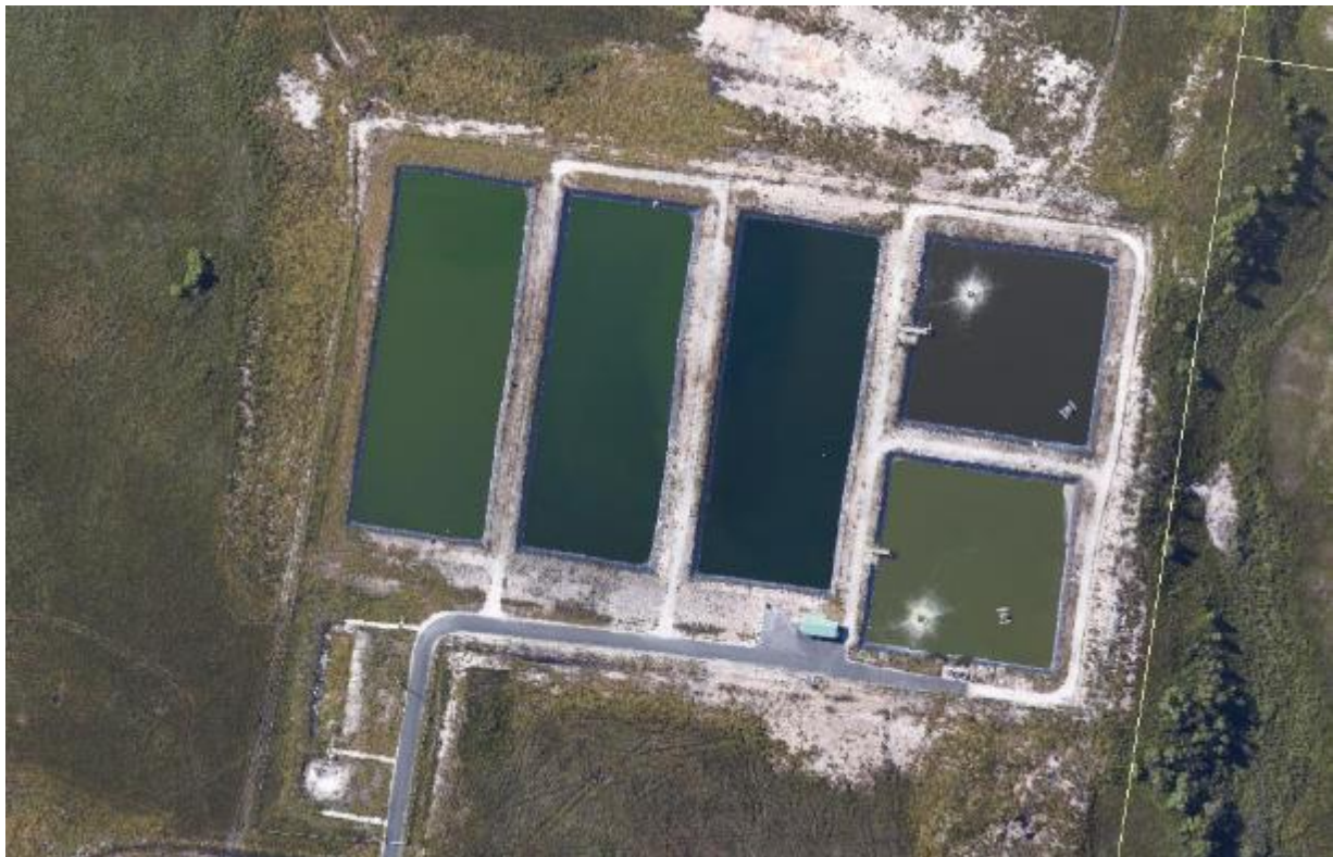
Figure 67-1: Strahan Sewage Treatment Plant
