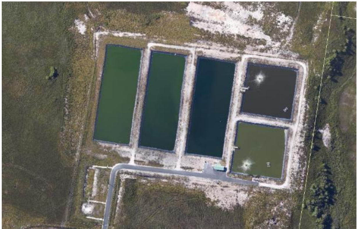
Figure 67-1: Strahan Sewage Treatment Plant
