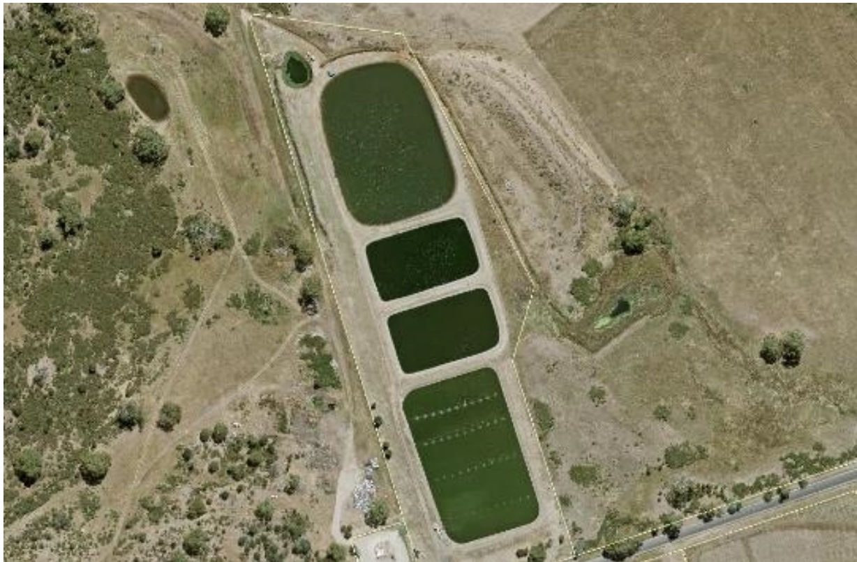
Figure 68–1: Swansea Sewage Treatment Plant
