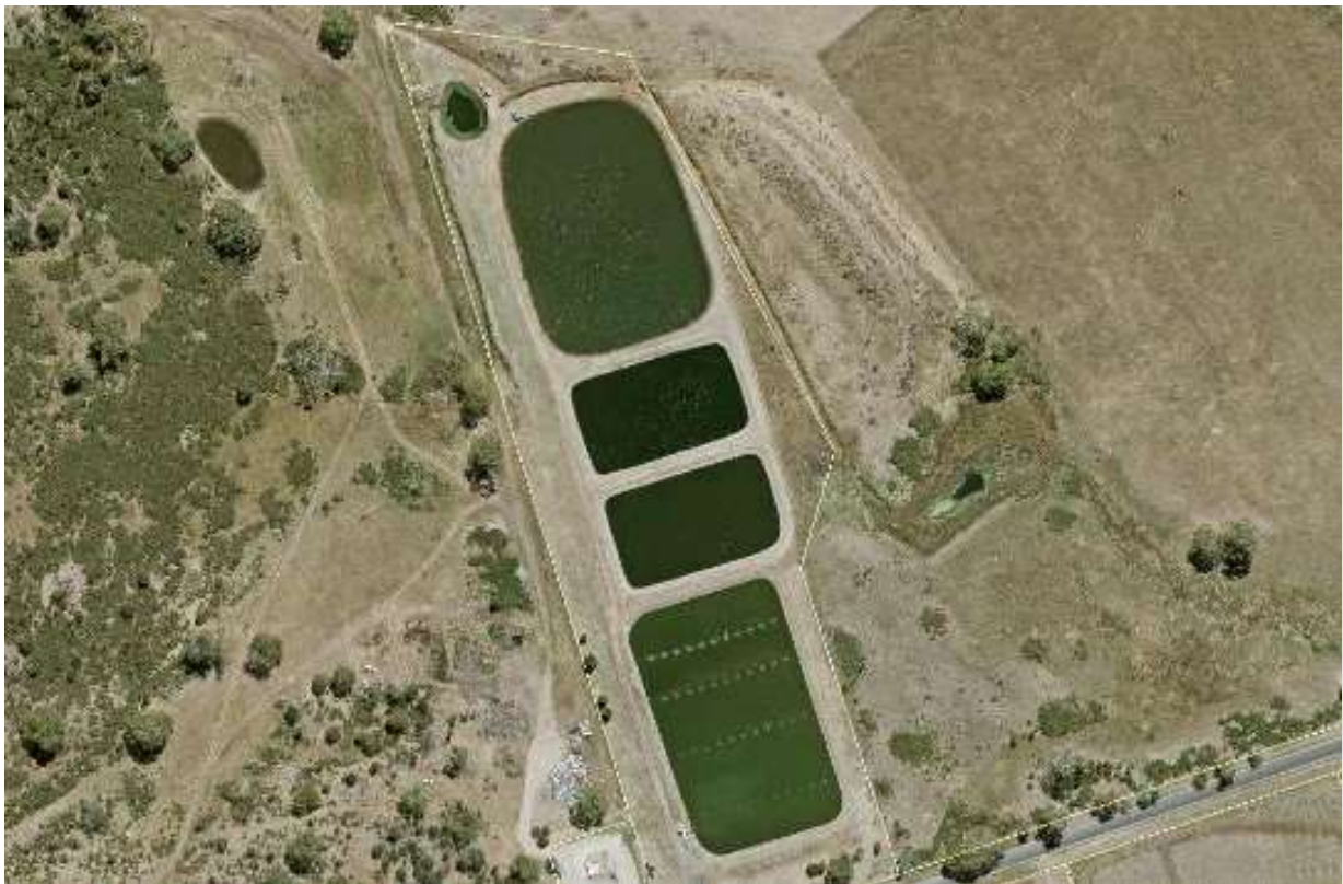
Figure 68-1: Swansea Sewage Treatment Plant
