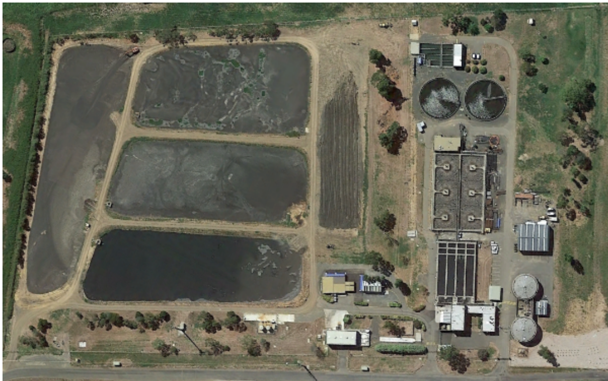
Figure 69-1: Ti Tree Sewage Treatment Plant
