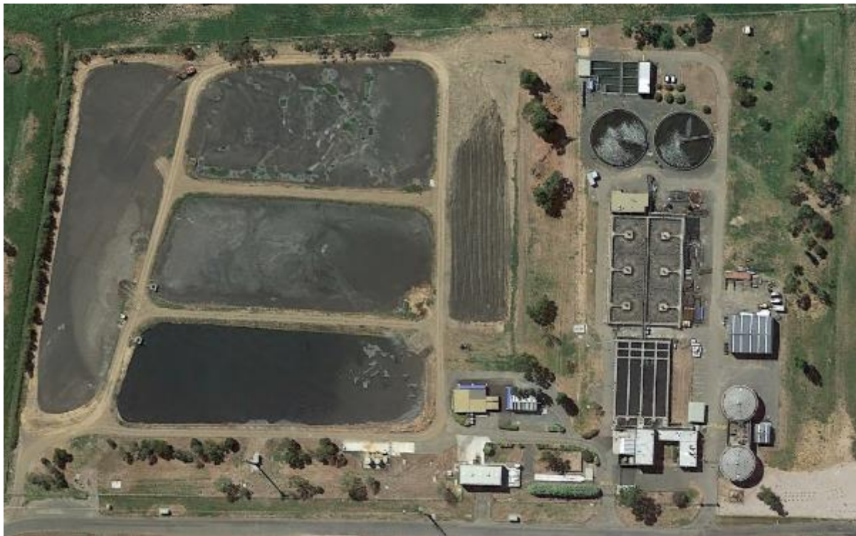
Figure 69-1: Ti Tree Sewage Treatment Plant
