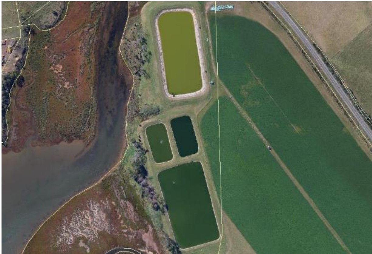
Figure 70-1: Triabunna Sewage Treatment Plant
