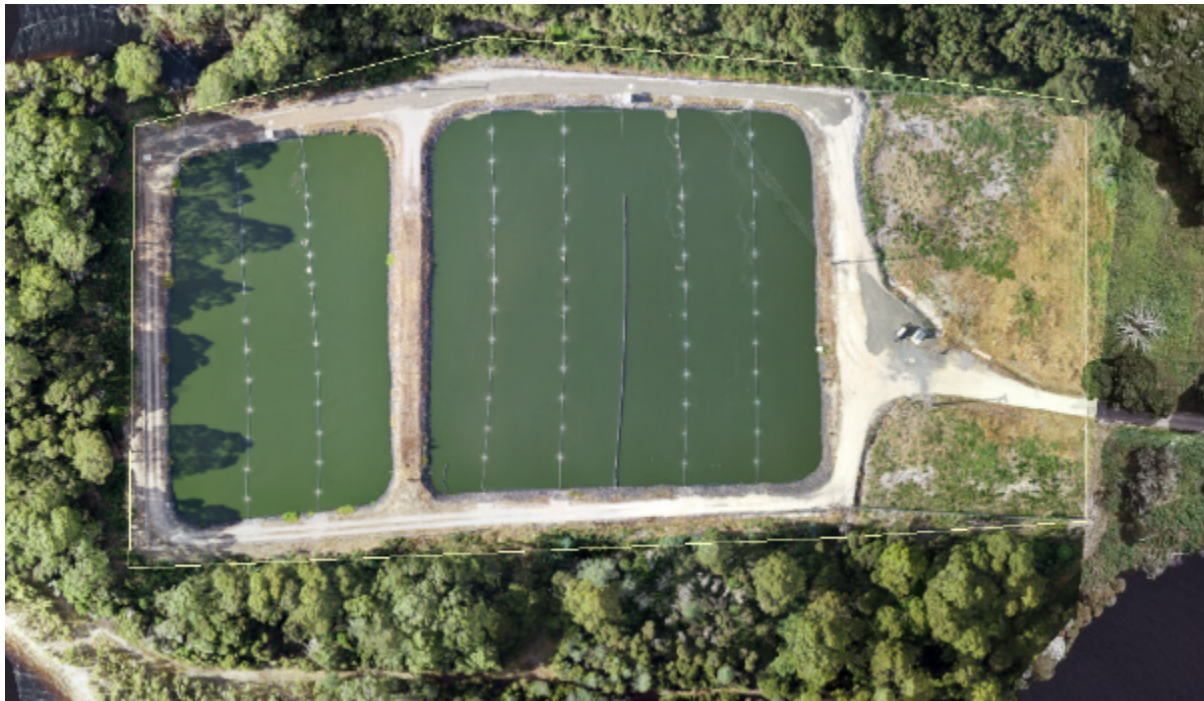
Figure 71-1: Tullah Sewage Treatment Plant
