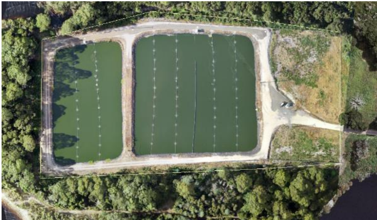
Figure 71-1: Tullah Sewage Treatment Plant
