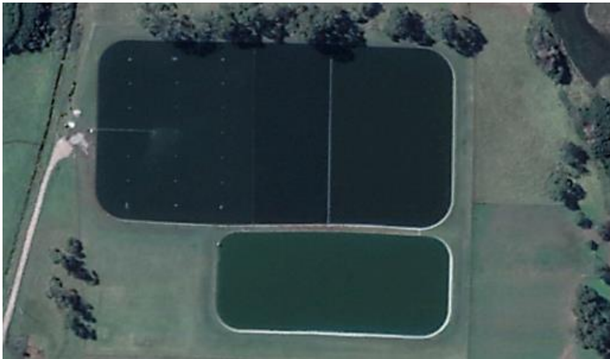
Figure 72-1: Turners Beach Sewage Treatment Plant
