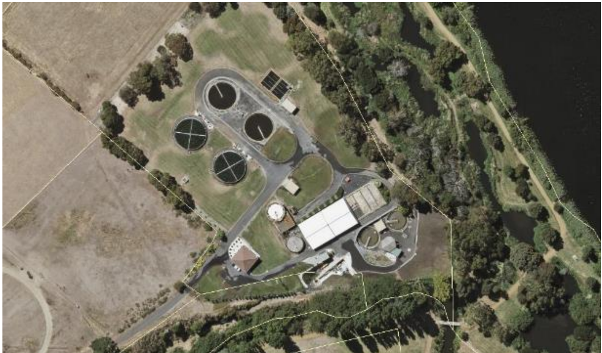
Figure 73-1: Turriff Lodge Sewage Treatment Plant
