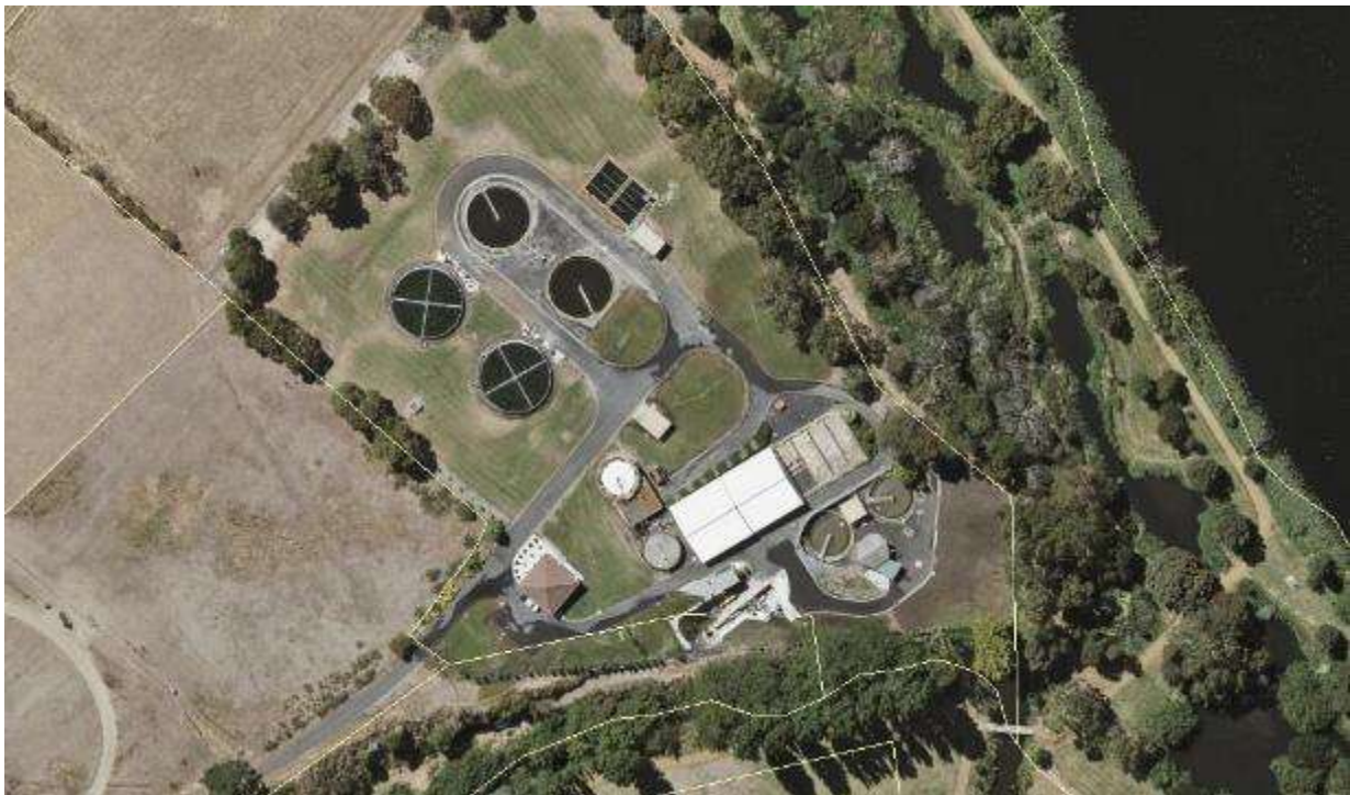
Figure 73-1: Turriff Lodge Sewage Treatment Plant
