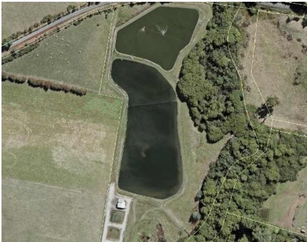
Figure 75-1: Westbury Sewage Treatment Plant
