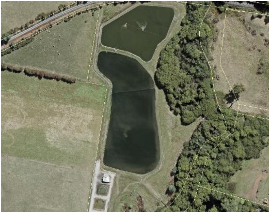
Figure 75-1: Westbury Sewage Treatment Plant
