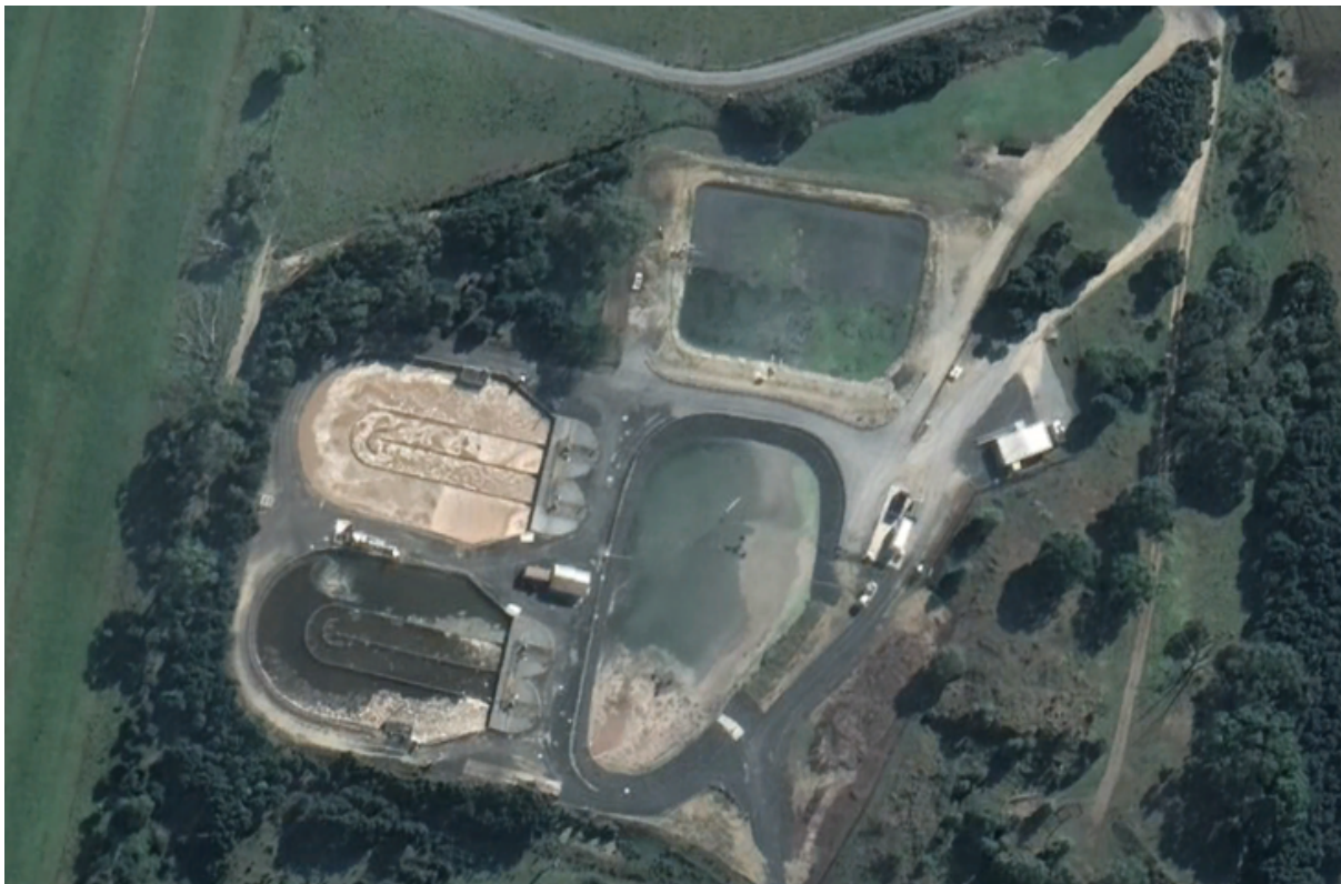
Figure 77-1: Wynyard Sewage Treatment Plant
