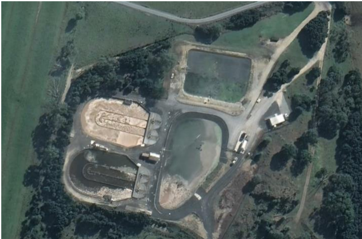
Figure 77-1: Wynyard Sewage Treatment Plant
