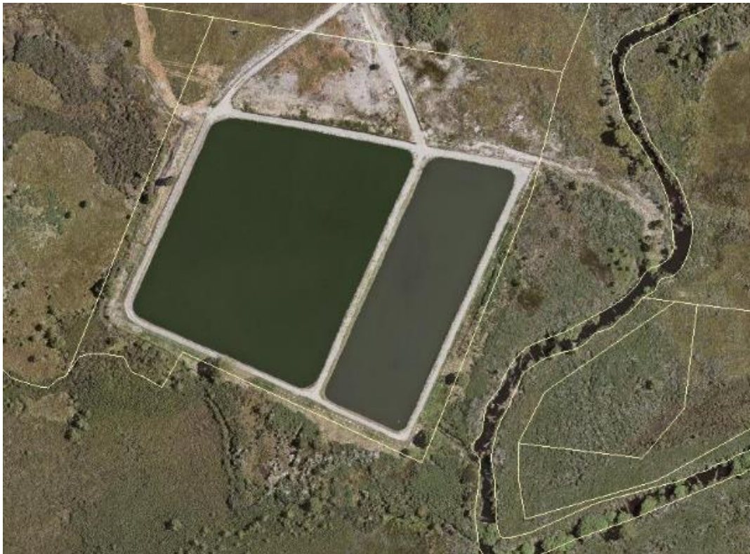
Figure 78-1: Zeehan Sewage Treatment Plant
