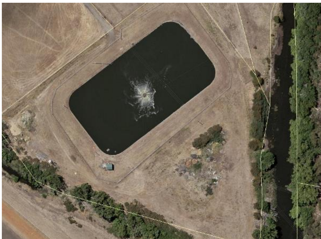
Figure 8-1: Brighton Sewage Treatment Plant
