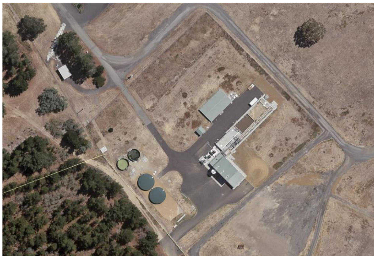
Figure 10-1: Sewage Treatment Plant
