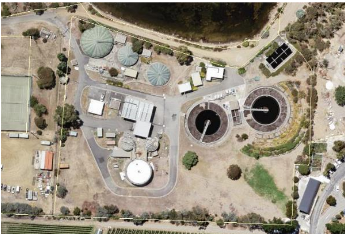
Figure 11-1: Cameron Bay Sewage Treatment Plant
