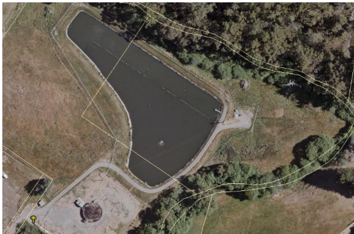
Figure 20-1: Dover Sewage Treatment Plant
