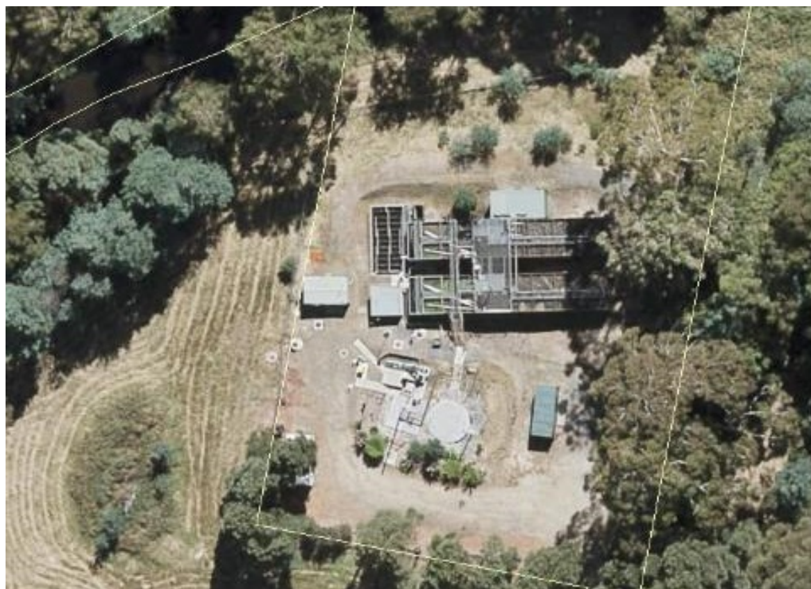
Figure 24-1: Geeveston Sewage Treatment Plant
