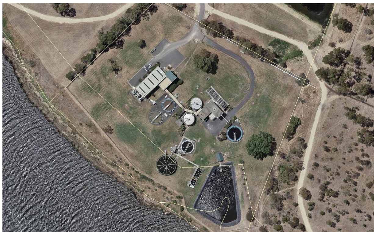
Figure 26-1: Green Point Sewage Treatment Plant
