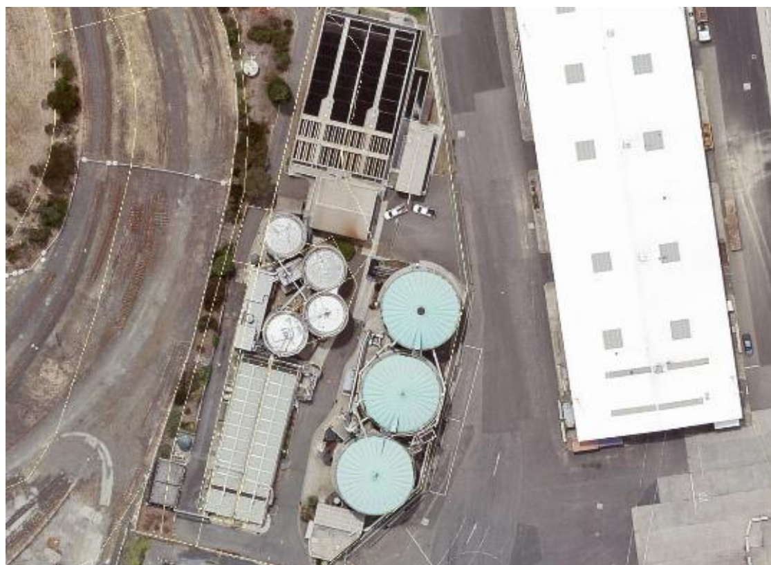
Figure 33-1: Macquarie Point Sewage Treatment Plant
