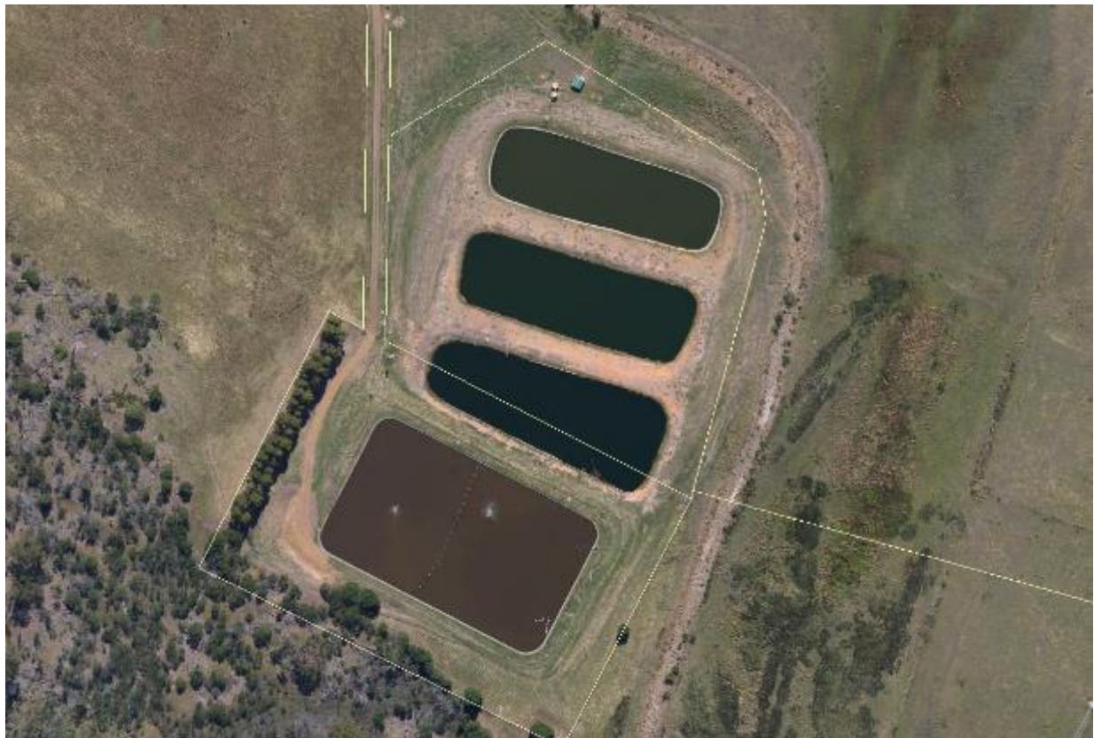
Figure 38-1: Orford Sewage Treatment Plant
