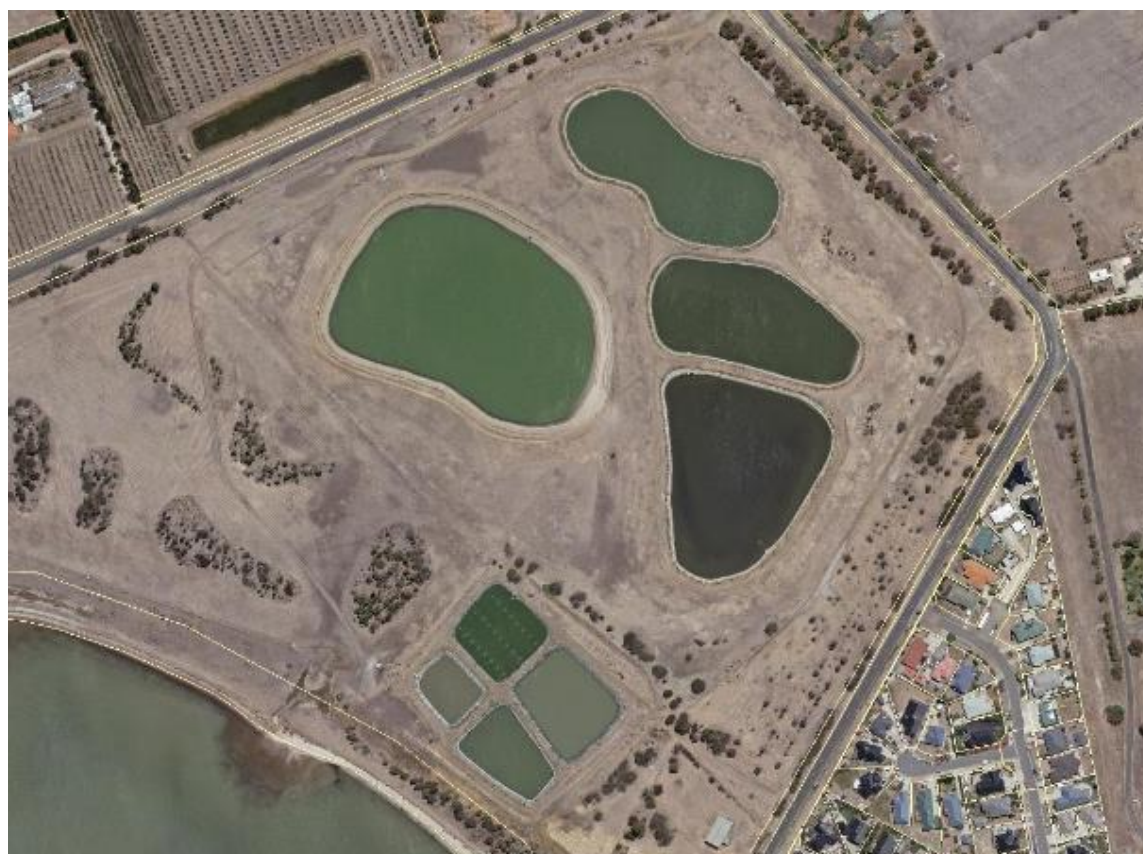
Figure 40-1: Penna Sewage Treatment Plant
