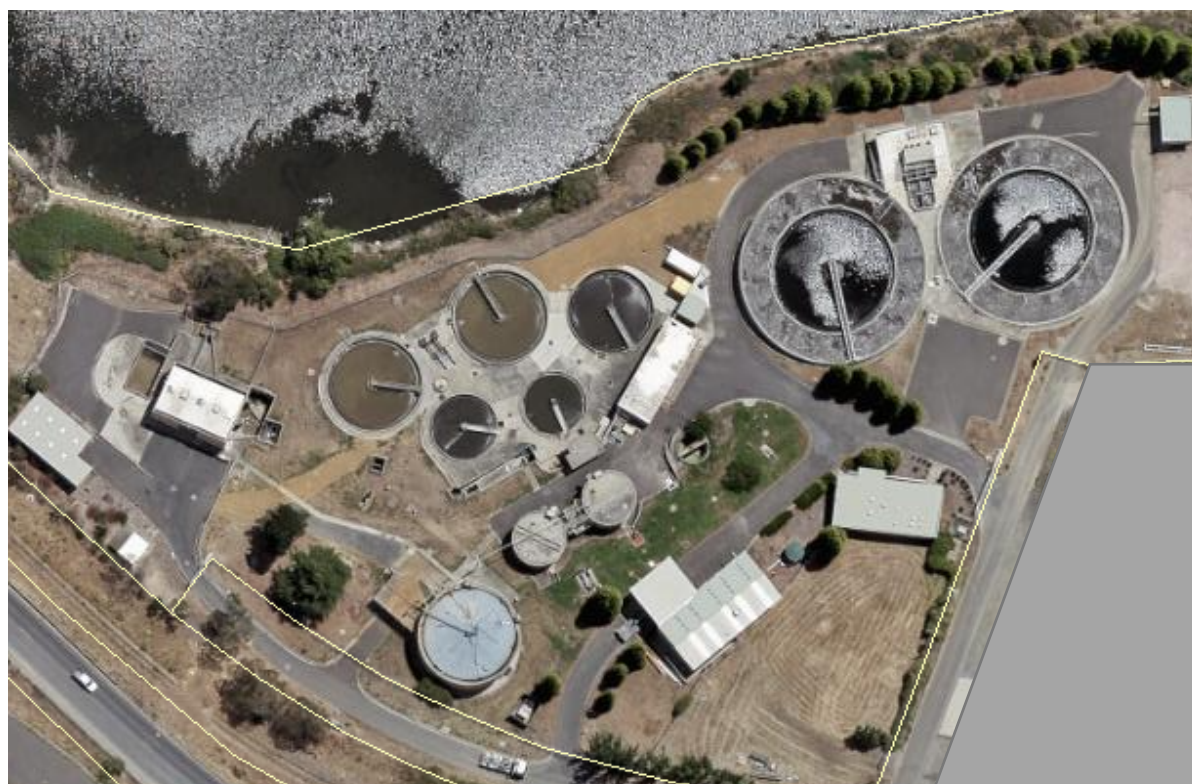
Figure 43-1: Prince of Wales Sewage Treatment Plant
