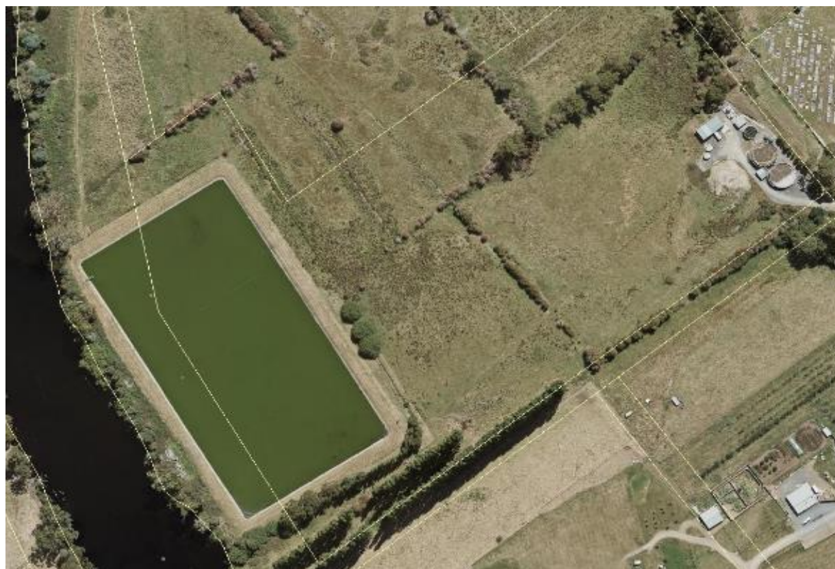
Figure 47-1: Ranelagh Sewage Treatment Plant
