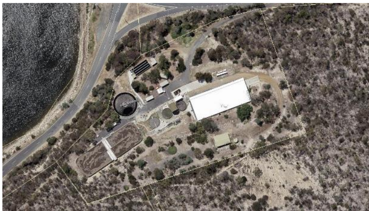
Figure 50-A: Risdon Sewage Treatment Plant
