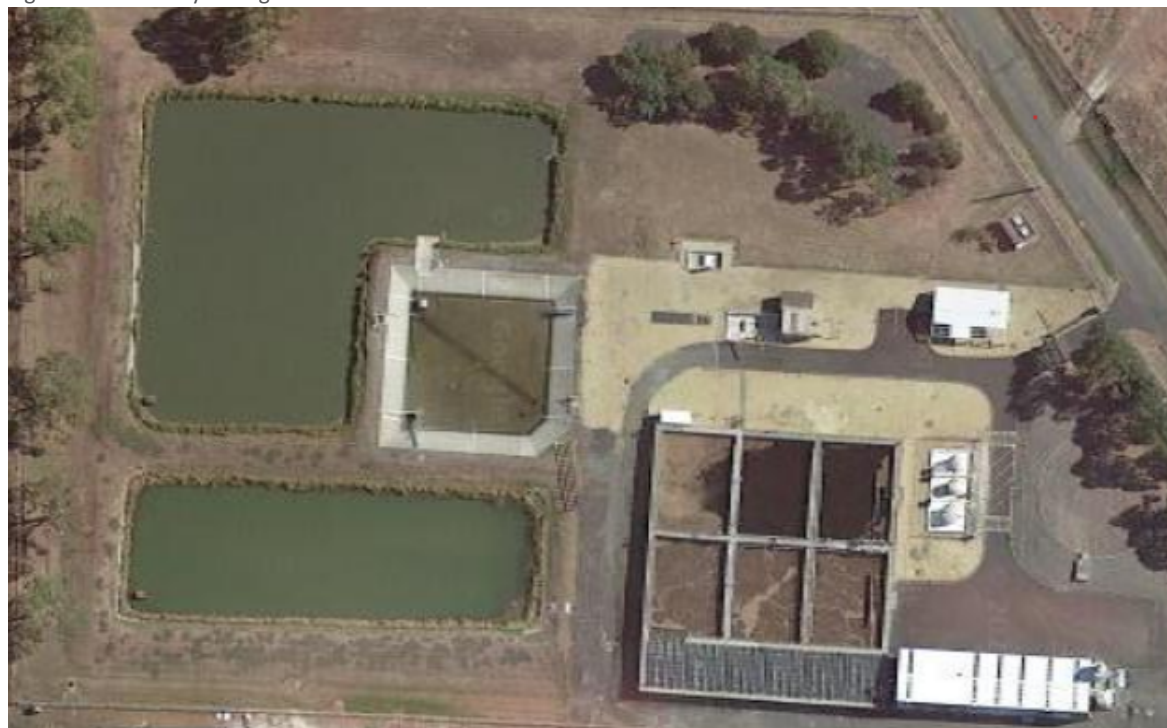
Figure 52-1: Rokeby Sewage Treatment Plant
