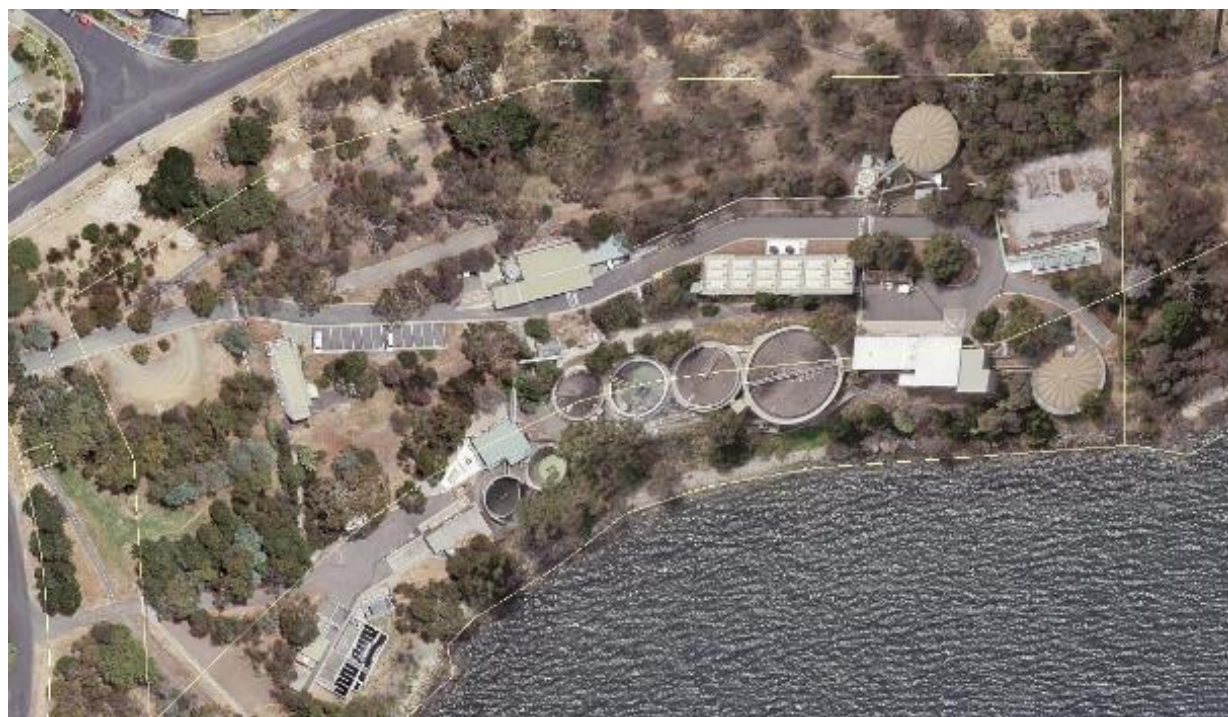
Figure 54-1: Rosny Sewage Treatment Plant
