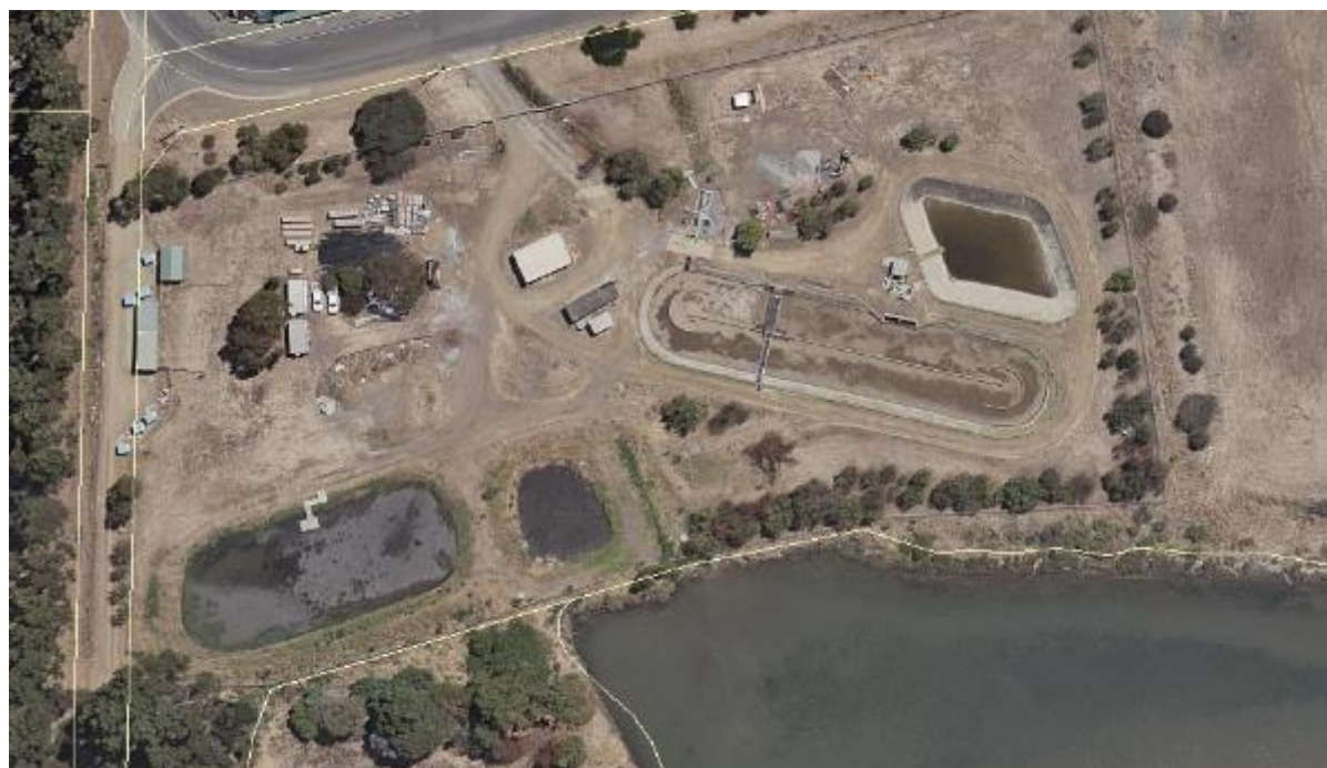
Figure 62-1: Sorell Sewage Treatment Plant
