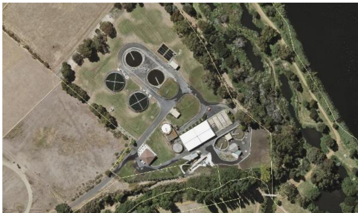
Figure 73-1: Turriff Lodge Sewage Treatment Plant
