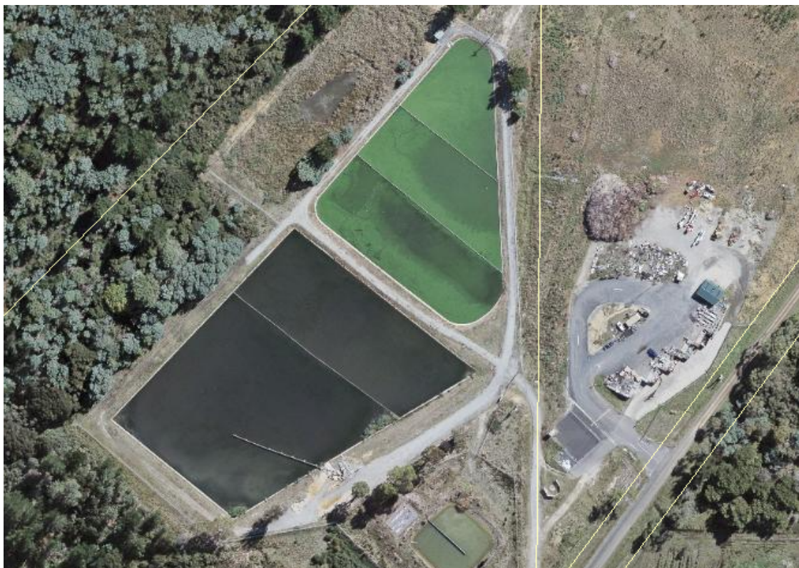
Figure 1-1: Beaconsfield Sewage Treatment Plant
