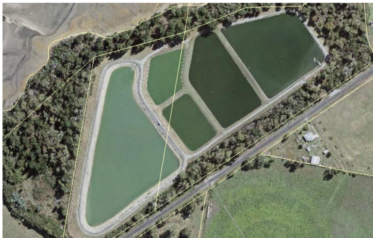
Figure 2-1: Beauty Point Sewage Treatment Plant
