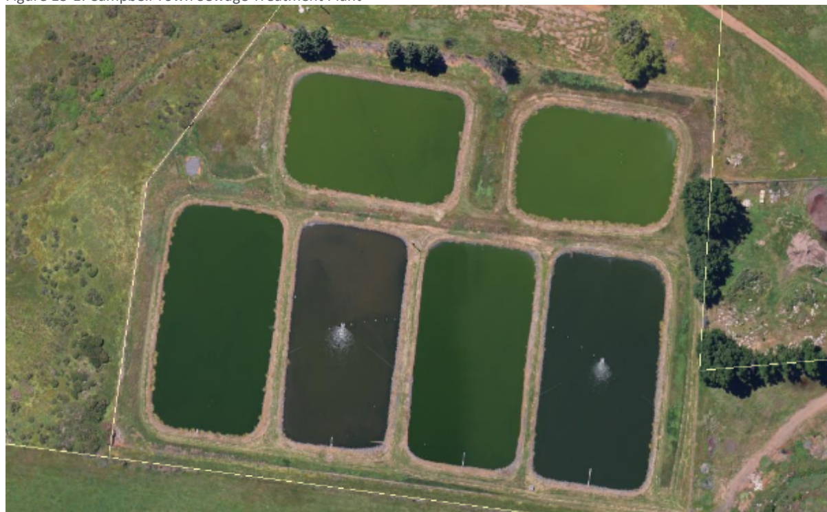
Figure 13-1: Campbell Town Sewage Treatment Plant
