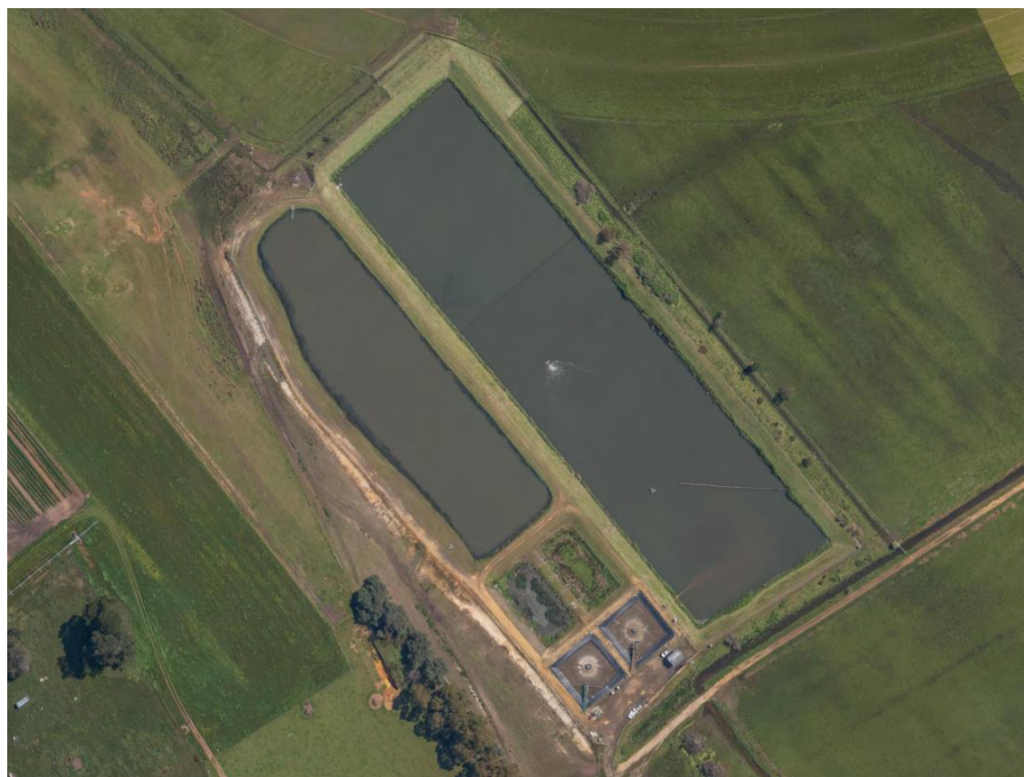
Figure 14-1: Carrick Sewage Treatment Plant
