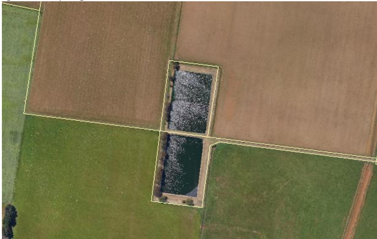
Figure 16--1: Cressy Sewage Treatment Plant
