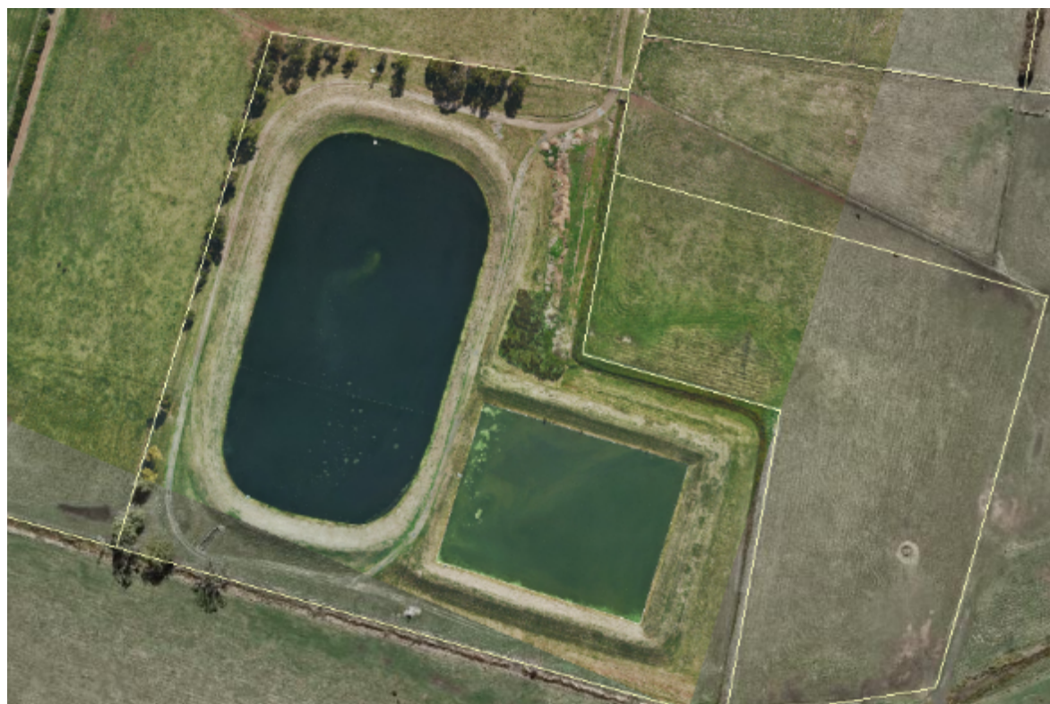
Figure 21-1: Evandale Sewage Treatment Plant
