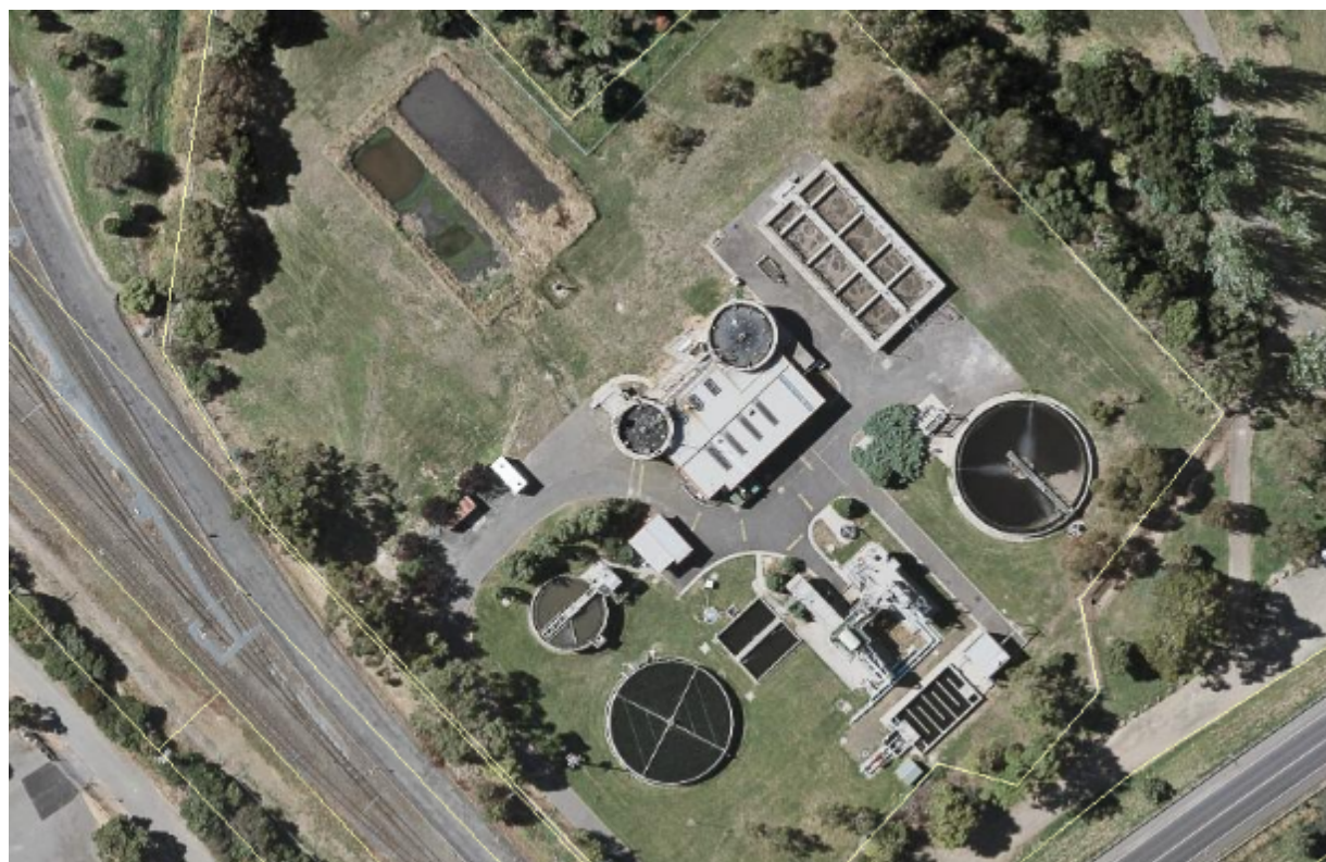
Figure 27--1: Hoblers Bridge Sewage Treatment Plant
